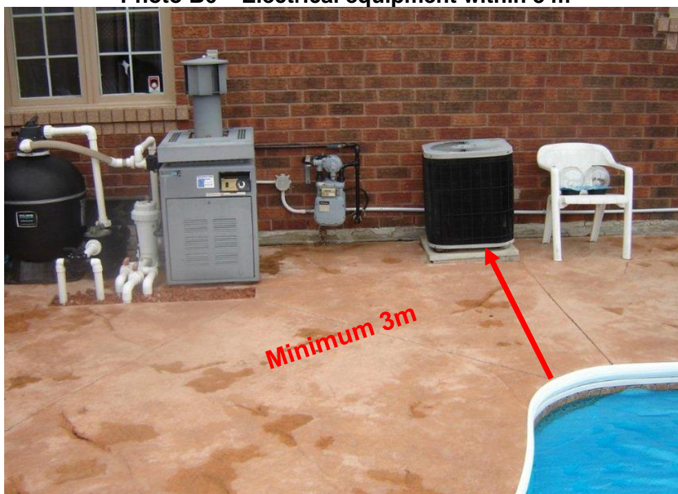
Photo B6 – Electrical equipment within 3 m
