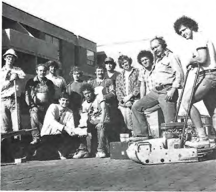
The Paving Stone Installers
