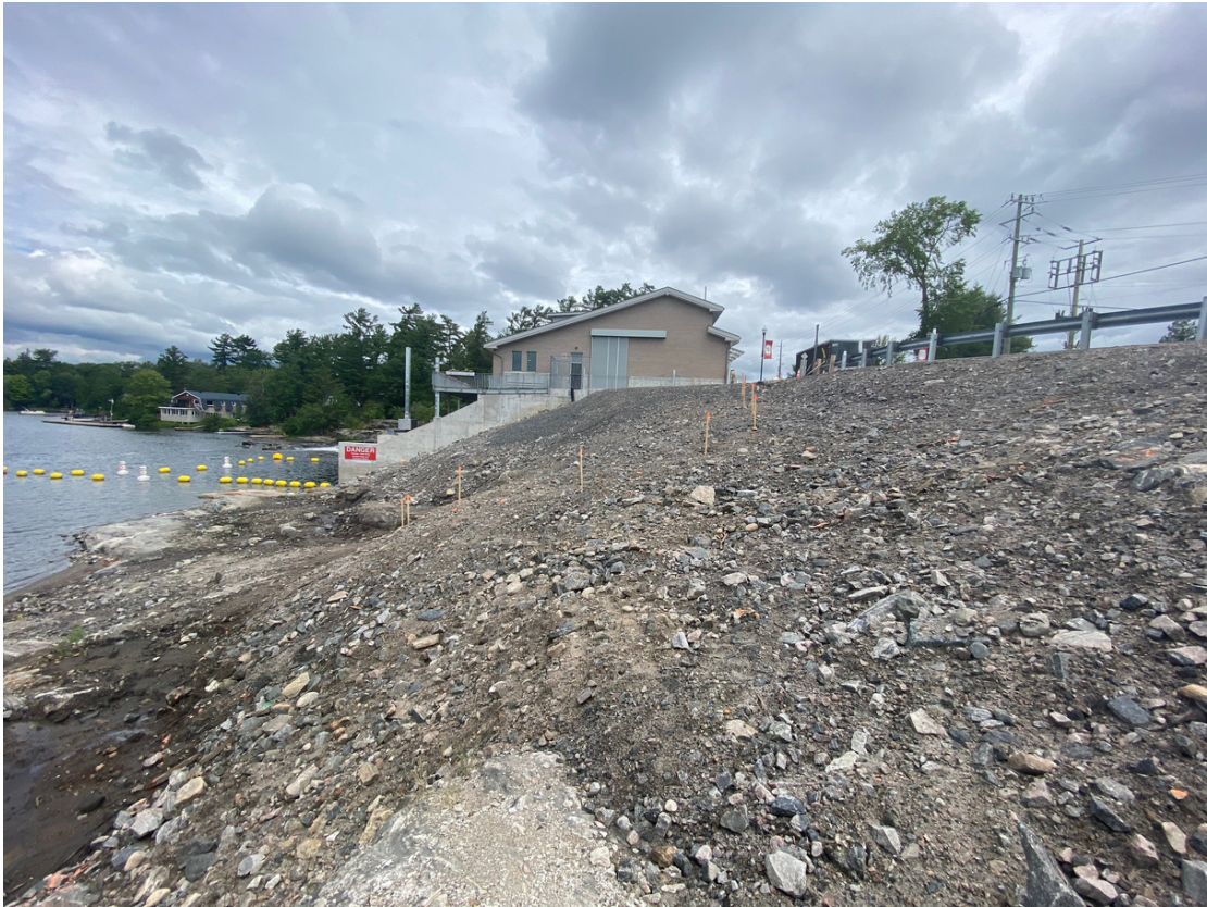
9. Site as of July 13, 2020. View from south
