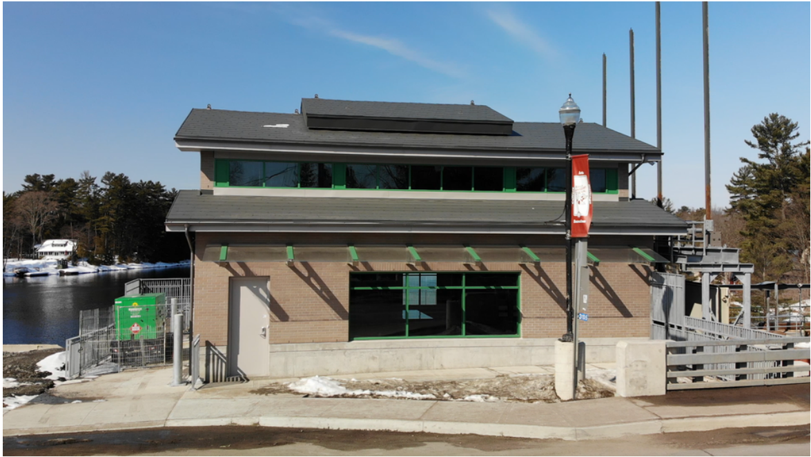
3. Front of Power House
