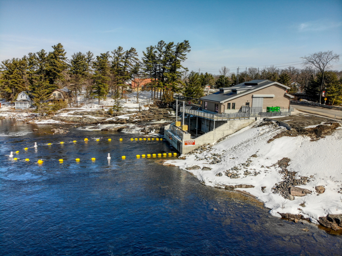
1. Power plant and park lands, looking towards north
