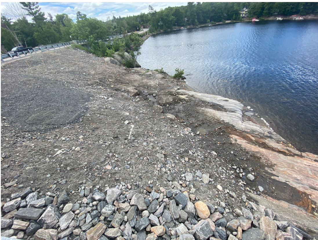
10. Site as of July 13, 2020. Looking downward toward water
