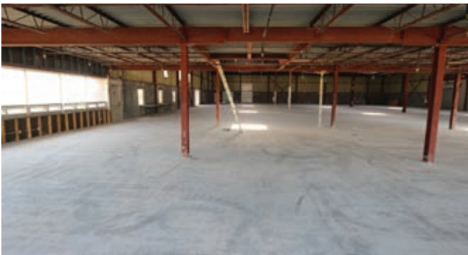
The building completely gutted.
